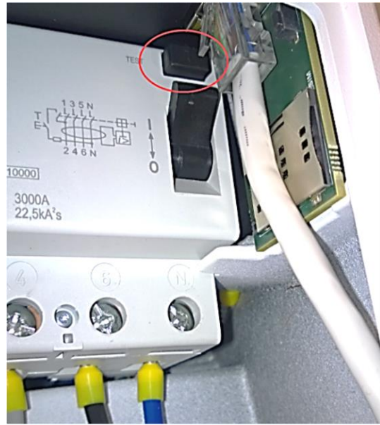
Figure 42: Bouton de test RCD
