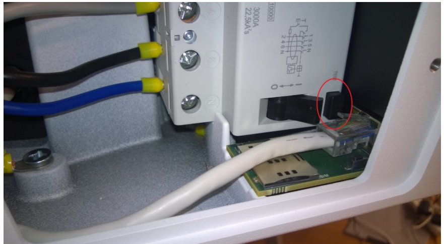
Figure 8: RCD test button
