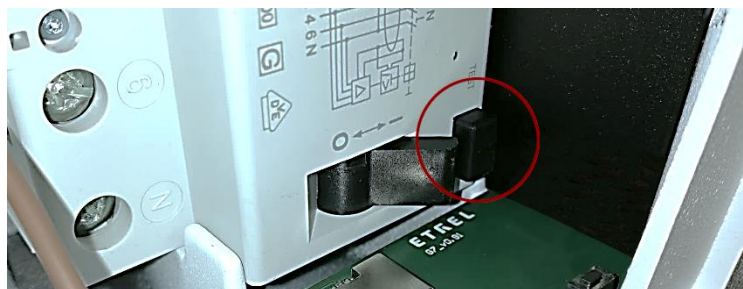
Figure 6: RCD test button
