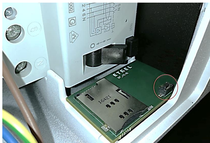
Figure 9: Reset button inside the maintenance opening
